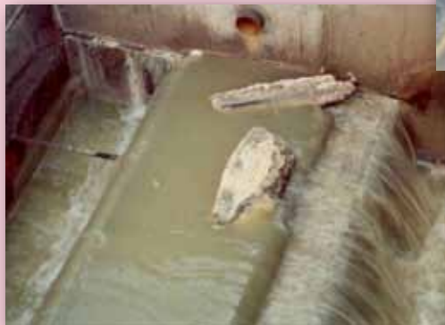
Above: Chunks of grease that arrived at the wastewater treatment plant.
