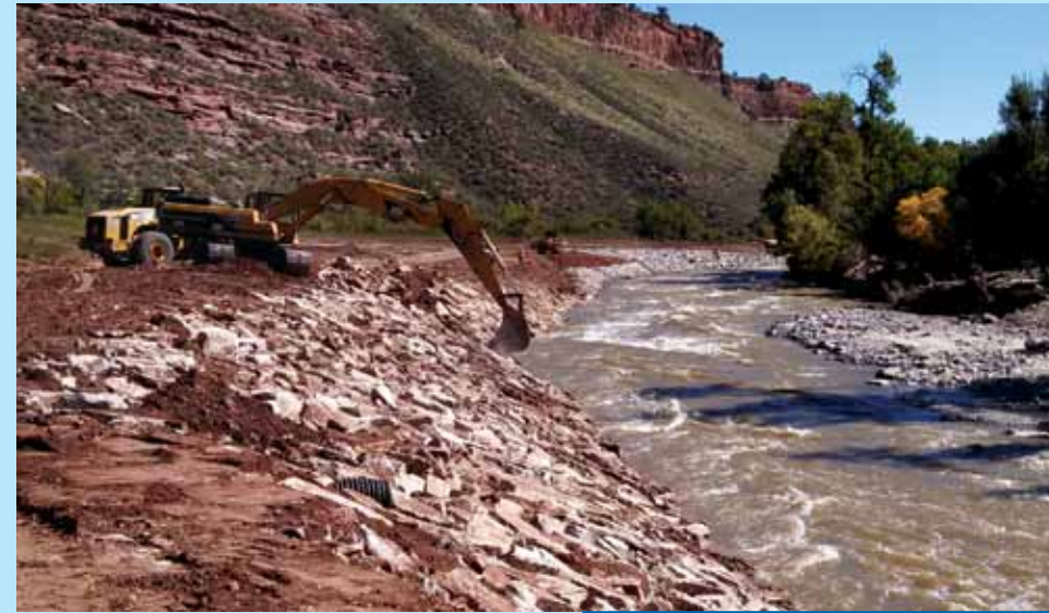
Crews worked to move the river back to its original path approximately two weeks after the flood last September. A new waterline, placed farther from the river than the two previous lines, will help the entire system be more resilient and resistant to damage from future floods.
