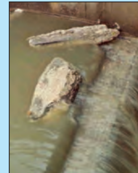
Hard chunks of compacted FOG arrive at the wastewater treatment plant.
