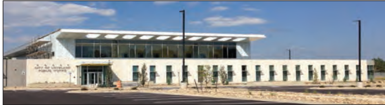
The south-facing main entry of the new service center, designed by the Denver office of global architectural firm RNL Design, features an unusual roofline that provides both shade and light.
