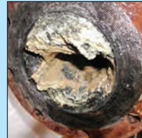
Clogged pipes in residences are the homeowner's financial responsibility.
