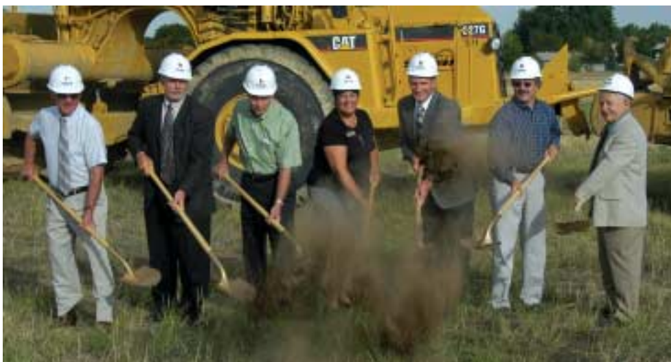
New beginning. Loveland City Councilors participate in a ceremonial groundbreaking for the new Fairgrounds Park project. The park, a complete renovation of the old county fairgrounds site east of Railroad Avenue, will include event pavilions, trails along the Big Thompson River, a skate park, ball fields, a dog park and more. Construction is expected to continue into autumn, 2008.
