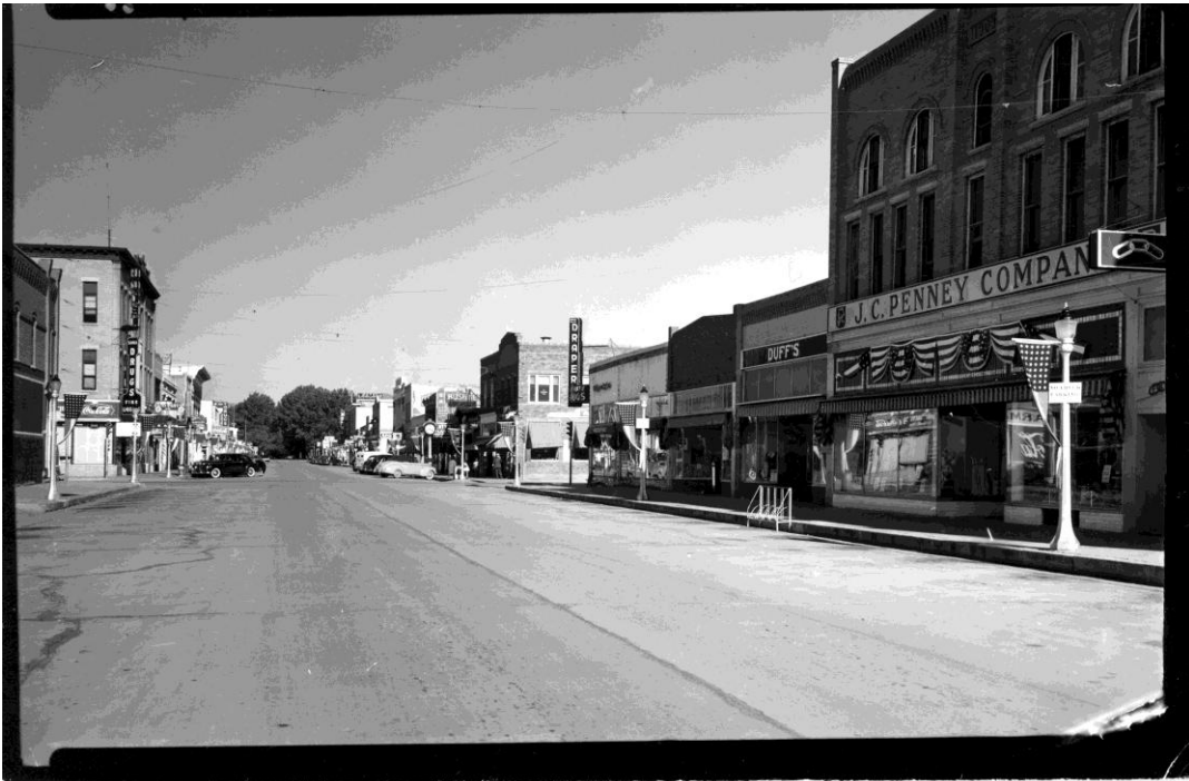
Picture 4: From the east, showing south elevation. c1969.
