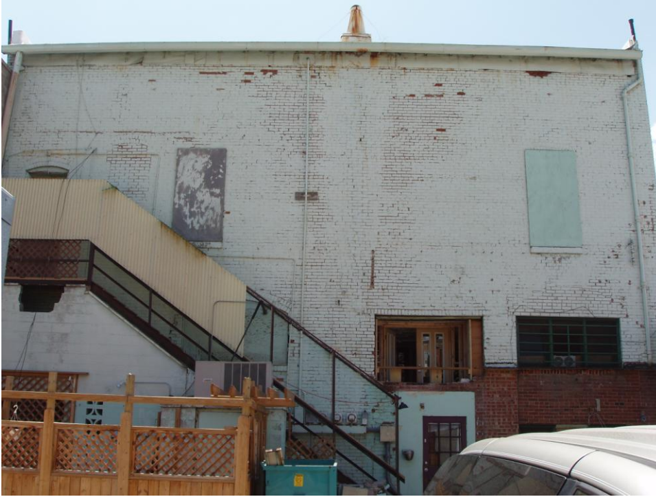
Picture 3: North elevation (rear).
