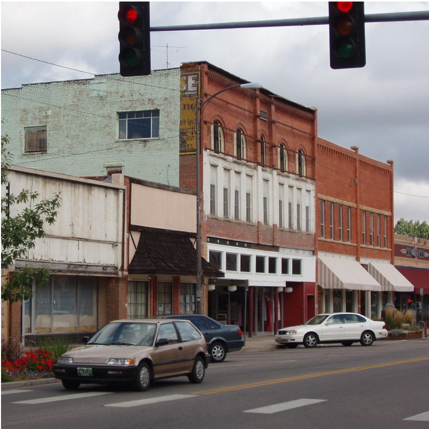
Picture 2: From the west showing the west and south elevations.
