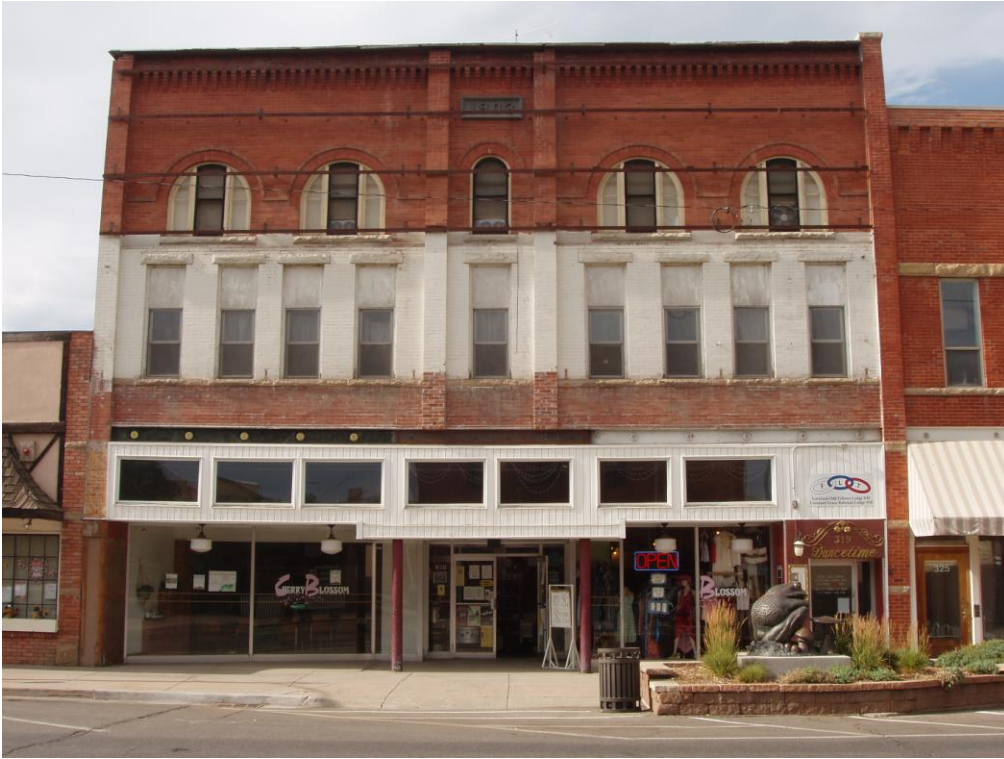
Picture 1: South elevation.
