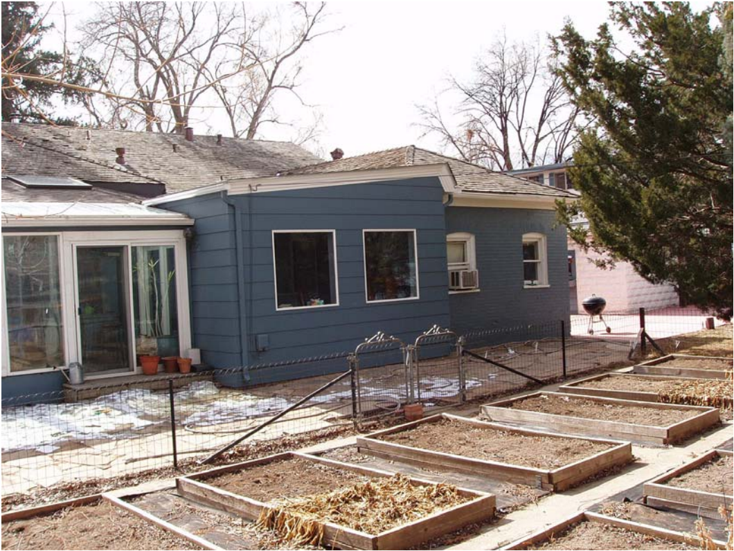
Northeast corner, west portion
