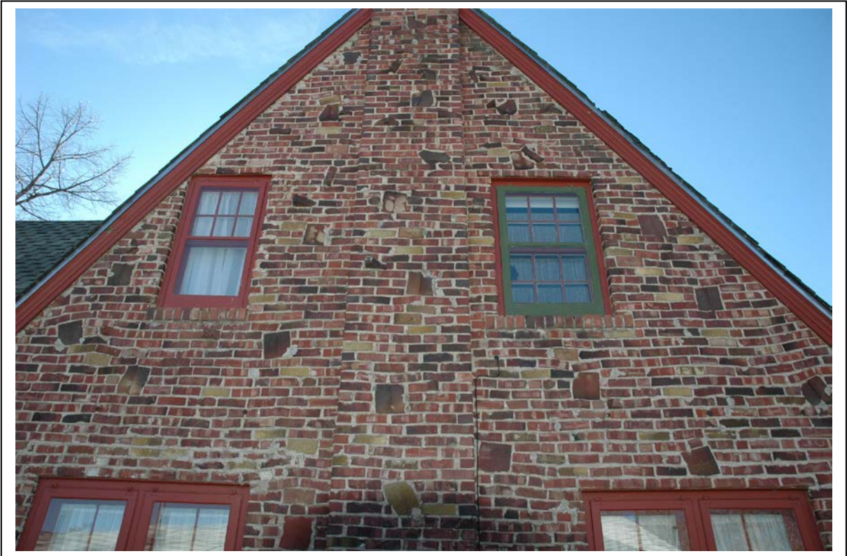
North Elevation – upper level
