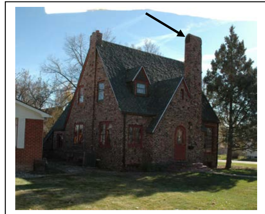
Photo No. 4 Main fireplace chimney with arching masonry cap.
