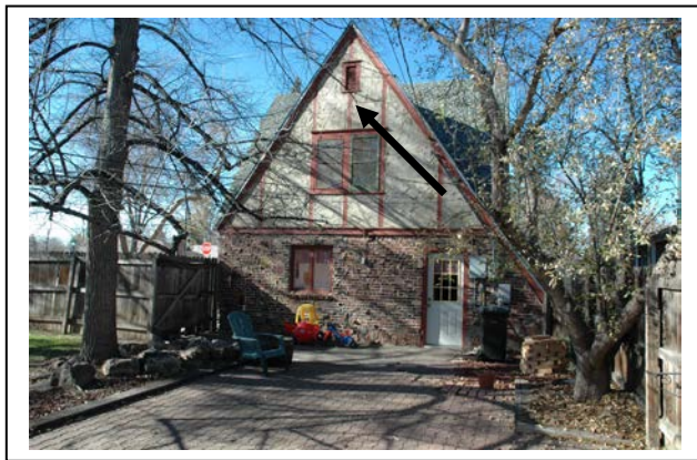
Photo No. 3 Example of typical half-timbering common to Tudor Revival style architecture.
