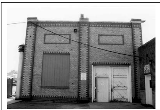
Photo 6. West elevation with former garage bay now featuring standard entry door.
