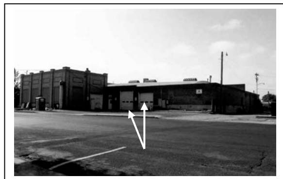
Photo 7. North elevation shows two garage bay entrances with modern roll-away doors.
