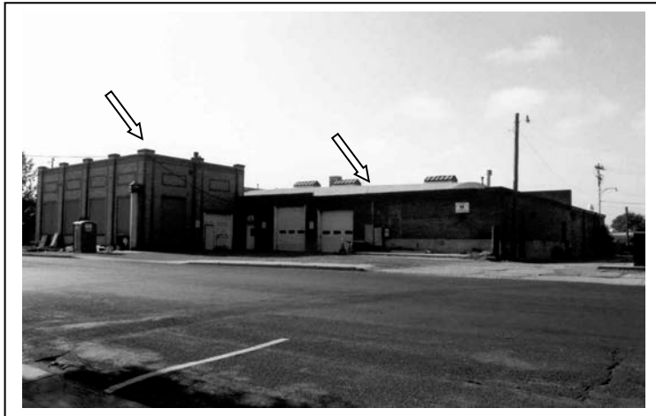
Photo #3. Two-story and one-story section of 451 Railroad/City of Loveland building.
