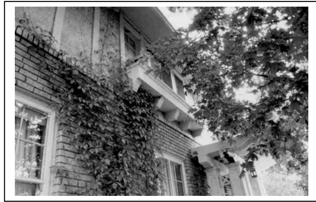
PHOTO #6 – Decorative window boxes, 8/1 and 6/1 double hung sash windows.
