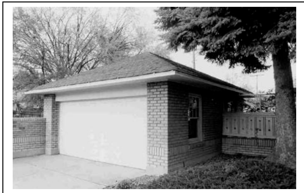
PHOTO #7 – Garage with connected brick garden wall. Wood fence panels with diamond shape motif.
