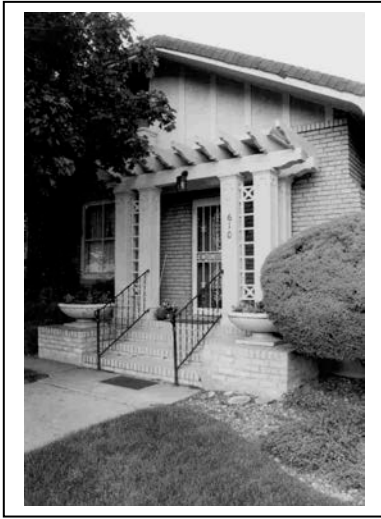
PHOTO # 5 –Porch with pergola roof and wood columns. Clipped gable roof.
